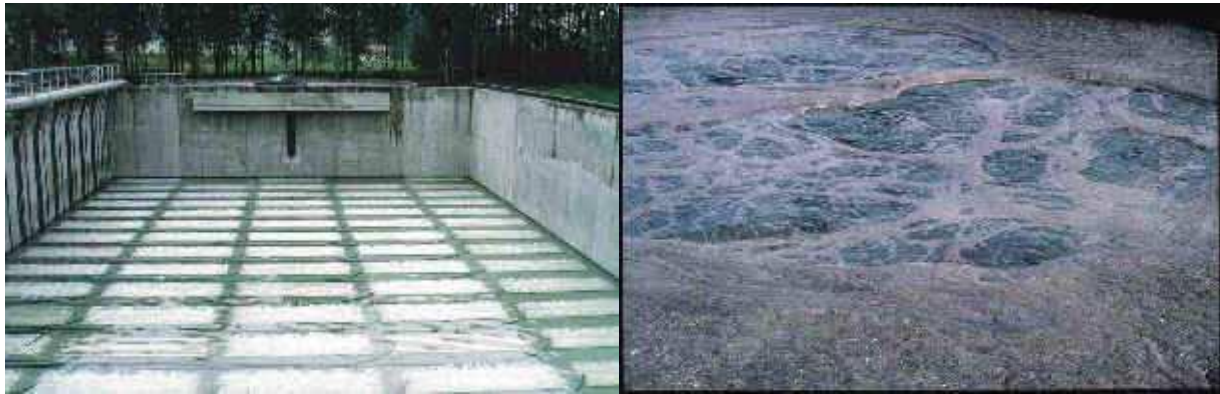
Picture 1. Nitrification tank before (left) and after (right) start-up
