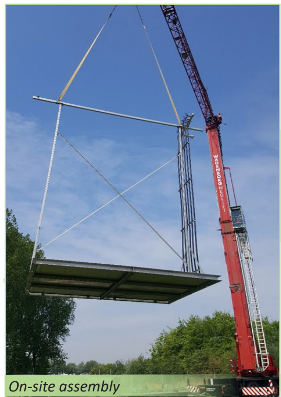
Frame with 6 mounted plate aerators
